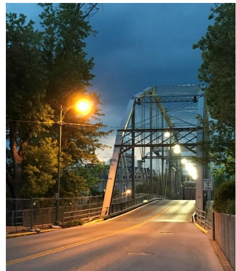
Figure 14: Bridge LED lights and conventional street lights.
