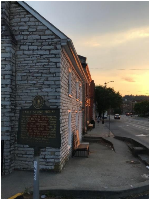
Figure 11: Historic building in Downtown Frankfort.
